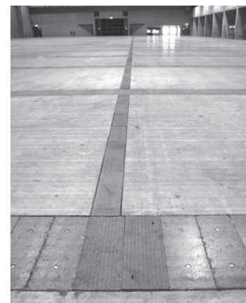
Pit and Sub-pit
