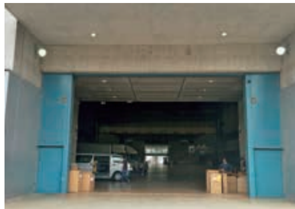
When move-in/out entrance is open
